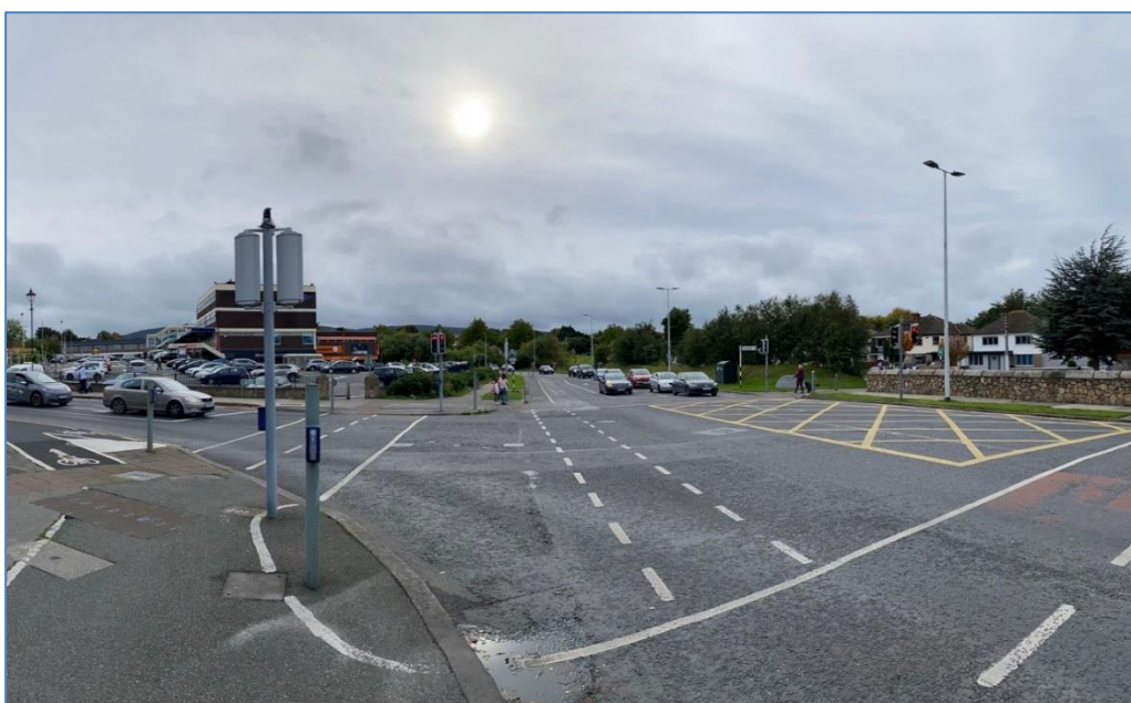
Figure 14.5: View showing the context between the northern end of the site (shopping centre car park to the left) and Sweetmount Avenue residential street (dwellings visible to the right)
