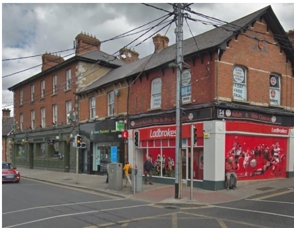
Ladbrokes/ Haven Pharmacy, Ryans Public House 54-57 Main Street
