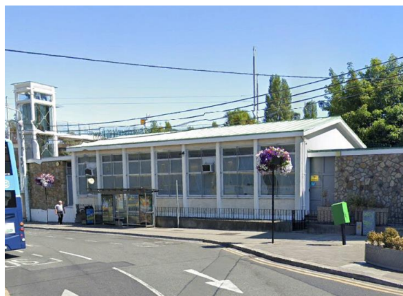
EIR Telecom Exchange, Main Street
