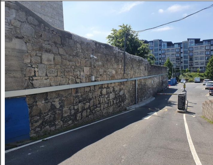
3. Northern Boundary Wall with Parochial House
