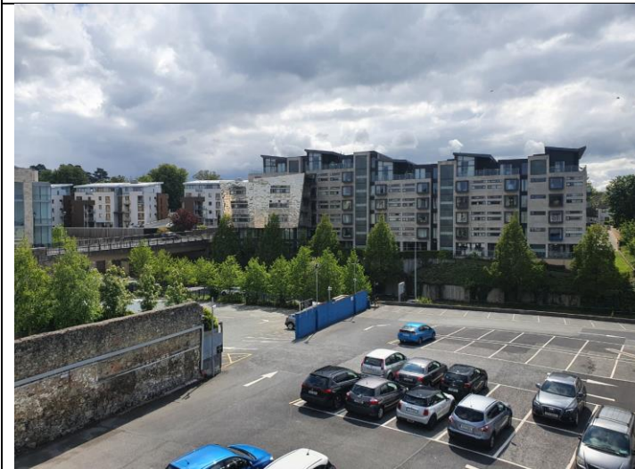
2. Car Parking at Rear of Former Mulvey's Hardware
